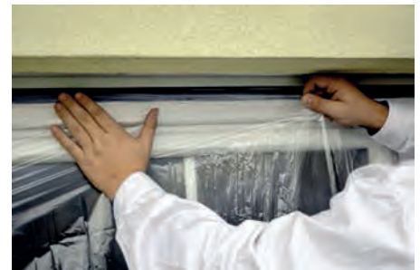
Apply dust sheet directly over tape
